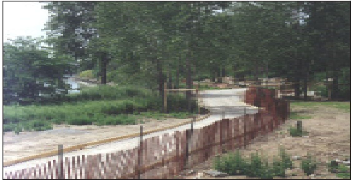
Site preparation for the new multi-use waterfront path in Soundview Park
