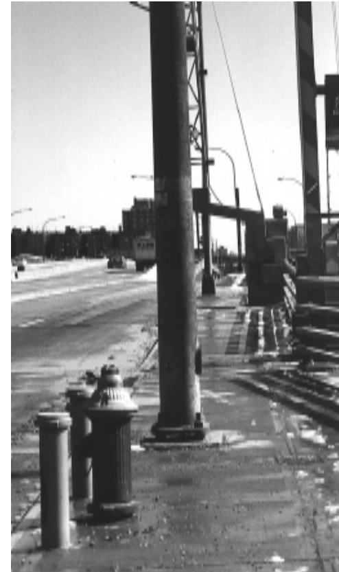
Eastern Boulevard Bridge, looking east
