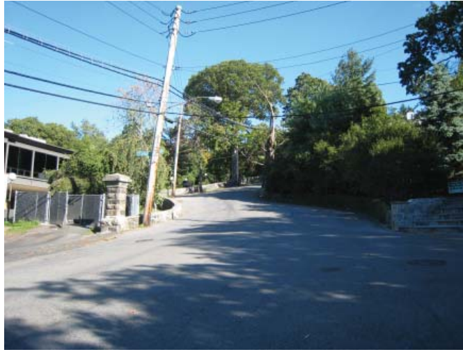
View of steep hill along W. 254th St. facing east
