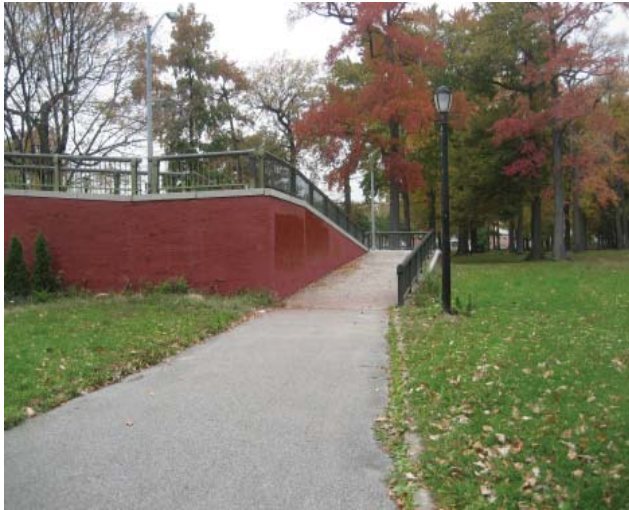
Buhre Avenue overpass east of Bruckner
