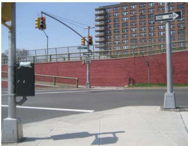
Roberts Avenue overpass, Middletown Road east of Bruckner.
