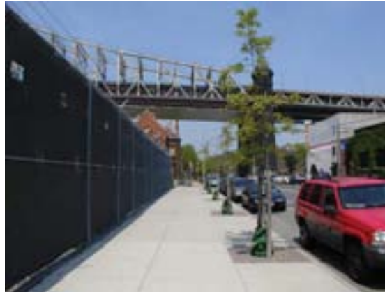
15-foot sidewalk along temporary power plant
