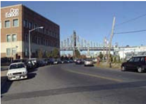
Vernon Boulevard at ConEd training facility
