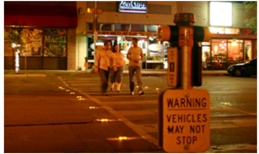
*IMAGE 17. A side view of embedded flashers. Image used with permission from John Wright of Dallas Voice.*
