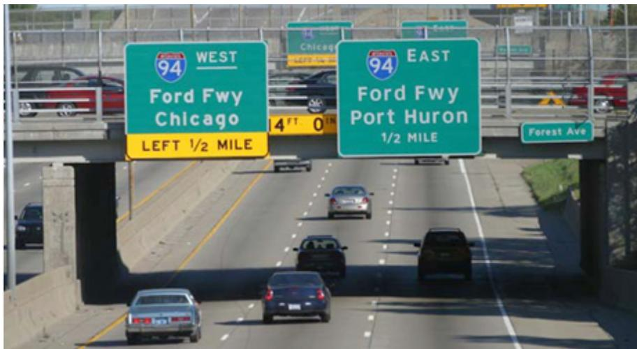
IMAGE 1. The difference can be seen in the fonts and the words East and West. The sign on the right is in Clearview font and the E in East is 25% larger than the rest of the word. Image used with permission from Michigan DOT.
