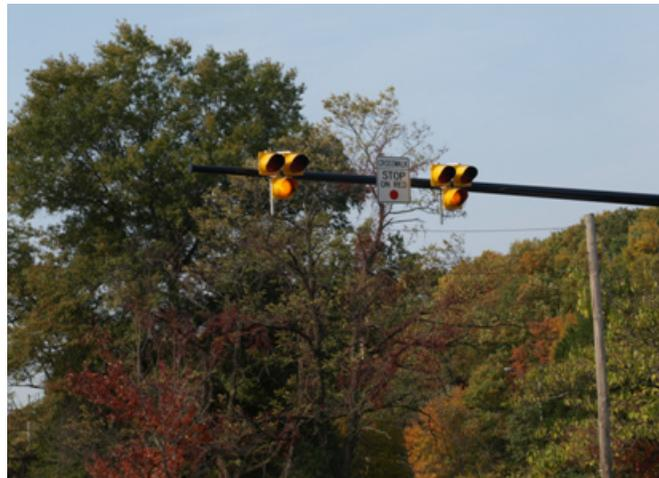
*Image 16. A flashing beacon installation. The amber light flashes on and off for a specified amount of time after the pedestrian passes through the bollard at the crosswalk's curb cut. Image used with permission from William F. Yurasko.*
