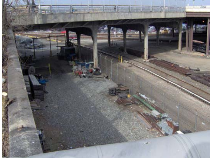
Parcel S0101 looking east. The bus terminal is to the right.
