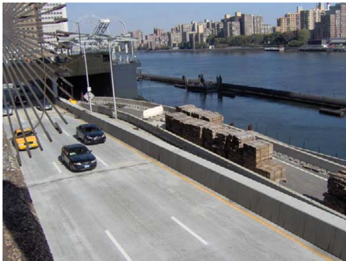
Parcel M0410, looking north from East 59 th Street
