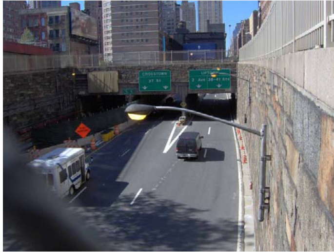
Parcel M0302, looking west from East 37 th Street (at far right) towards 2 nd Avenue
