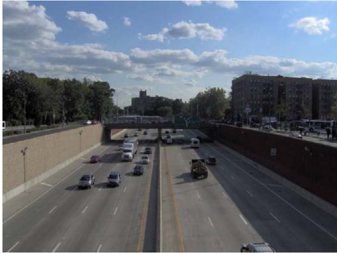
Parcel B0701 looking south from pedestrian overpass towards Wilkinson Avenue.
