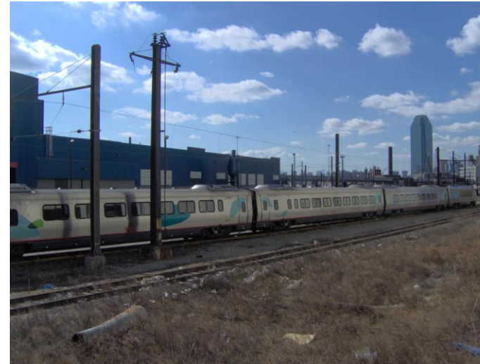
Amtrak's service and inspection building (at left in photo) would break the plane of a deck over parcel Q8007, Sunnyside Yards.
