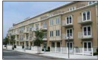
Row-house on Rockaway Beach Blvd. in the proposed R5D in Rockaway Beach
