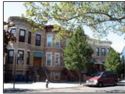
Row houses on 64th Place within a proposed R5B district in western Glendale
