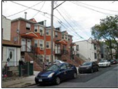
Out-of-character three-story attached buildings on 78th Avenue within an R5 district in western Glendale
