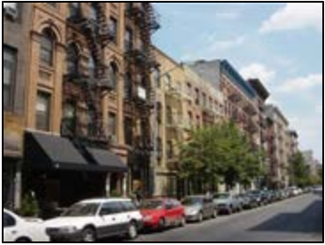
North side of East 2nd Street, between Avenue A and Avenue B
