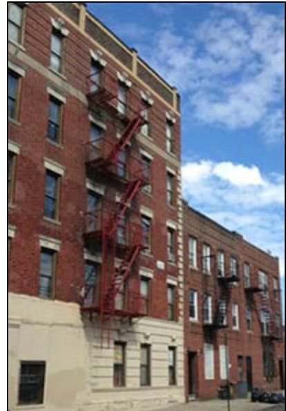
Apartment buildings on Beaumont Avenue & East 189th Street
