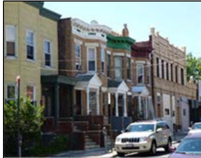
Row houses on Hoffman Street
