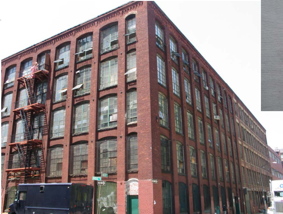
Water and Front St
