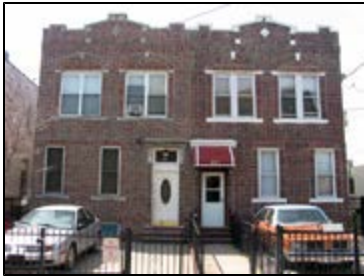
Semi-Attached Homes on the south side of 36th Street between 12th and 13th Avenues.
