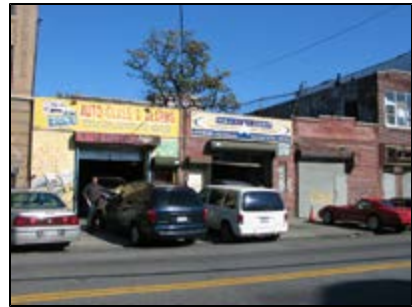
Proposed M1-2/R6B district on the north side of 39th Street between 12th and 13th Avenues.
