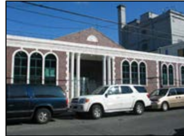
Community Facility use on 38th Street between 13th and 14th Avenues.
