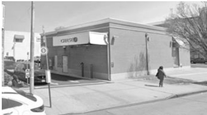
Blank walls along retail streets that create unwelcoming sidewalks
