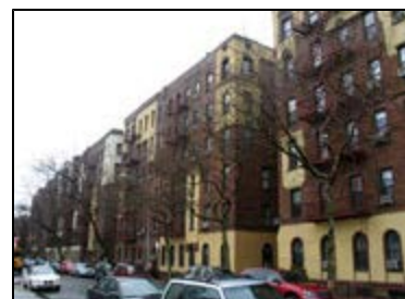
Typical character in the proposed R7A district on Brighton 12th Street between Corbin Place Ocean
