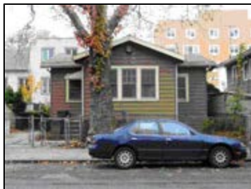
Single family home in the bungalow area on 5th Street between Ocean View Avenue and Neptune Avenue
