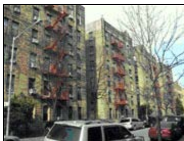
Multi-family apartment buildings on Brighton 12th Street between Ocean View and Brighton Beach Avenue
