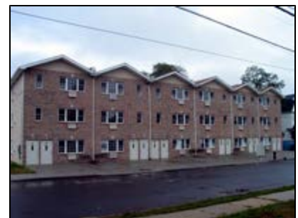
New out-of-character development in R5 District Nameoke and Gipson Streets
