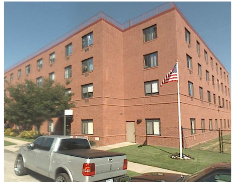
Castleton Manor Senior Housing, Staten Island
