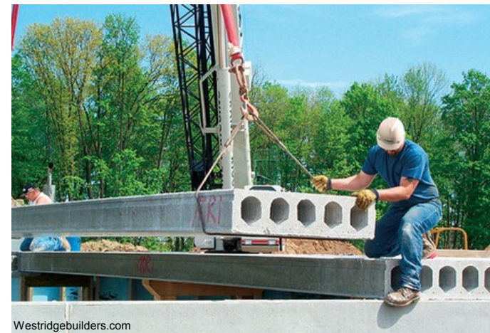
‘Block and Plank’ construction
