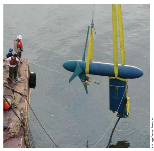
Installation of Verdant Power tidal turbines in the east channel of the East River.
