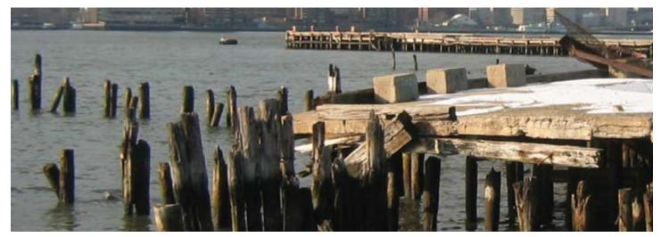
Without regular maintenance, piers will deteriorate until they collapse, as seen with this pier in Greenpoint, Brooklyn. It is difficult to obtain a permit to rebuild.
