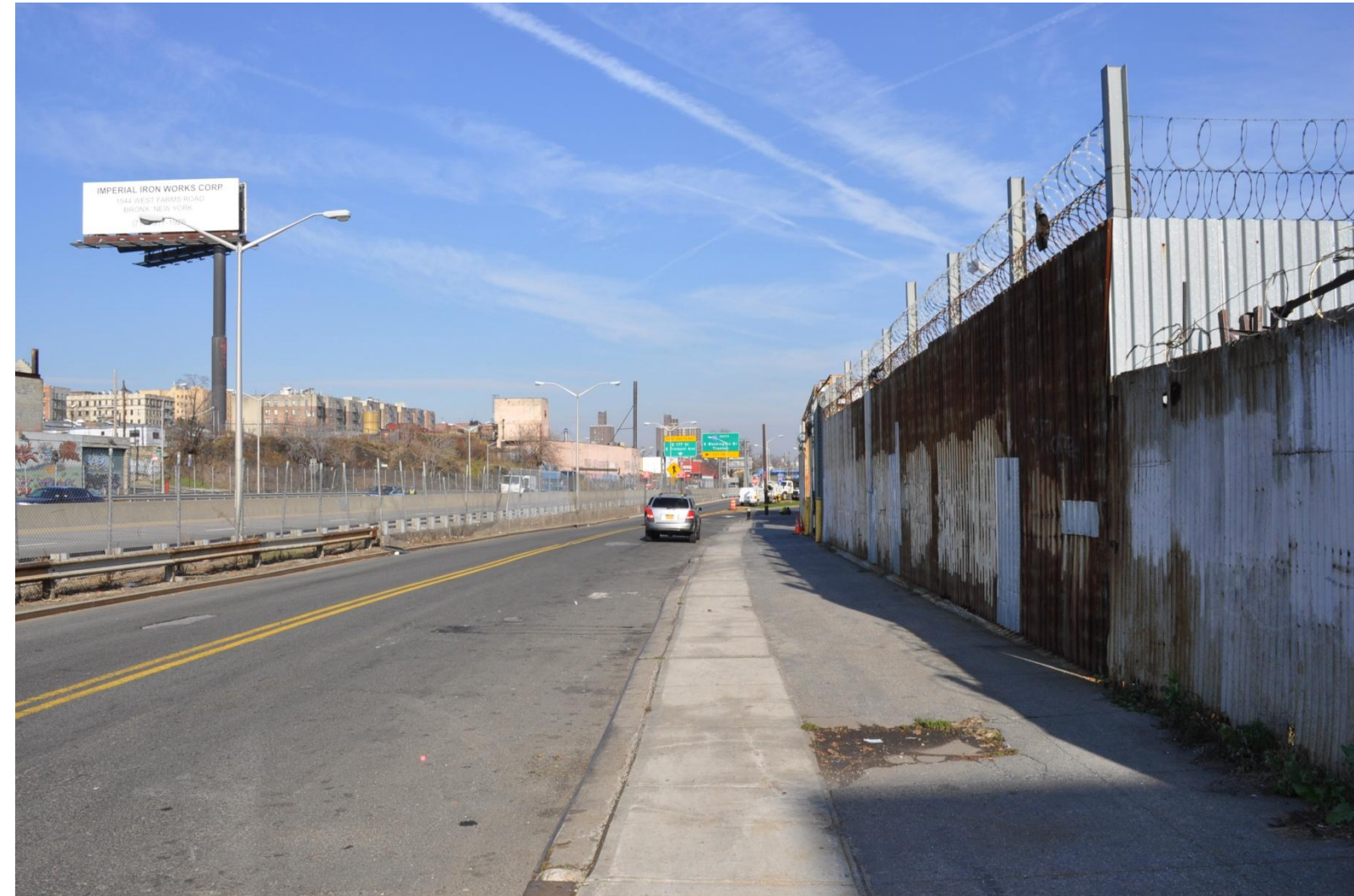
View south towards E 172 nd street
