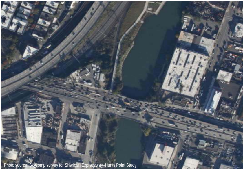
Photo source: Skidmore survey for Sheridan Expressway-Hunts Point Study Photo courtesy of NYCDOT
