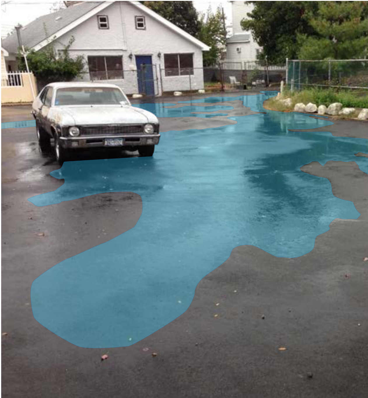
Stormwater sheet flow and ponding on surface parking areas in Harding Park.
