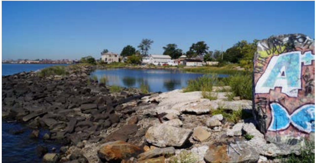
Breakwaters in Harding Park.
