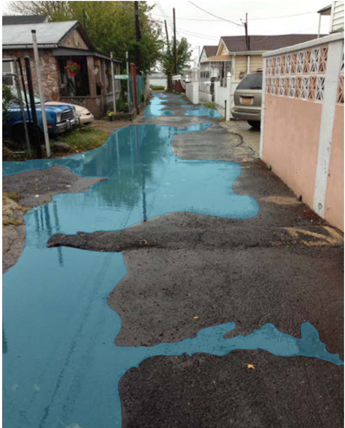
Stormwater ponding on private streets in Harding Park.
