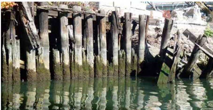
Deteriorating bulkheads
