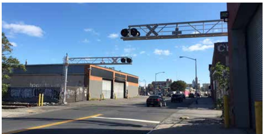
Rail crossing at Morgan Avenue
