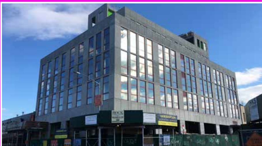
100 Bogart Street: new construction coworking space
