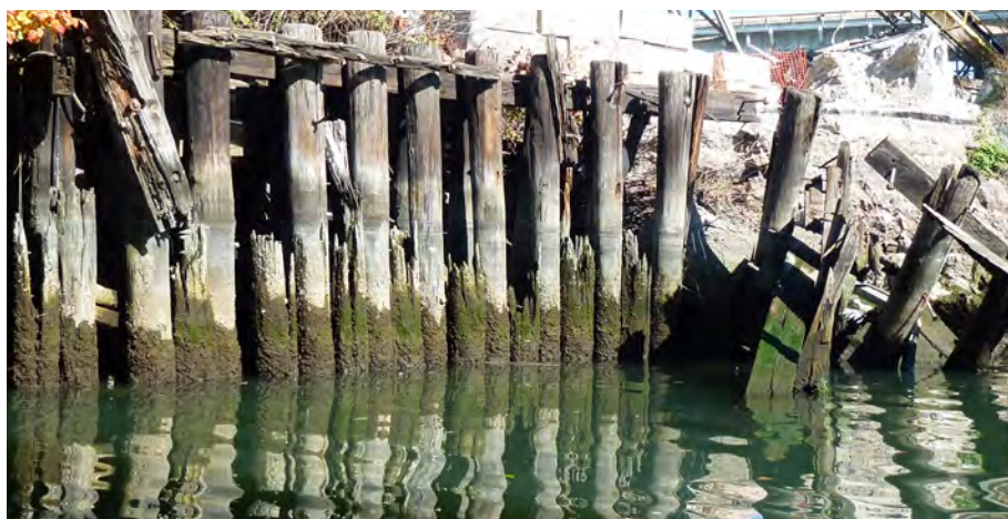
Deteriorating bulkheads
