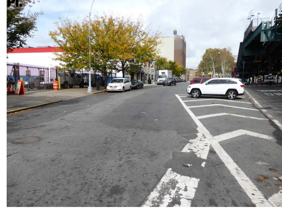
Confusing roadway with unsafe conditions for pedestrians and frequent vehicle speeding
