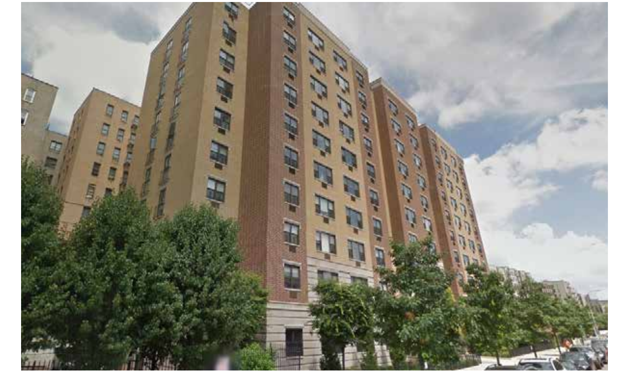
1275 Grant Ave. Completed 2010 | Terminado 2010
