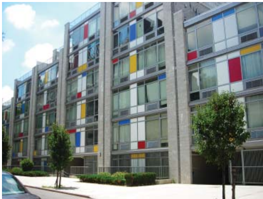
A six-story building on Spencer Street built between 1998 and 2008
