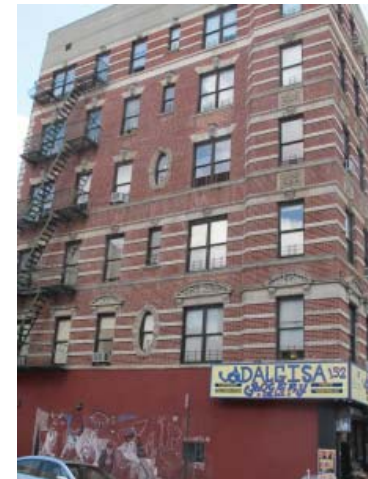
A six-story building on East 111th Street built before 1961
