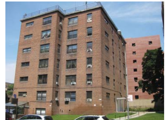
A six-story building on Dongan Avenue built before 1961
