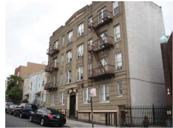
A four-story building on 19th Street built before 1961
