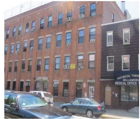
A four-story building (at left) on Metropolitan Avenue built before 1961
