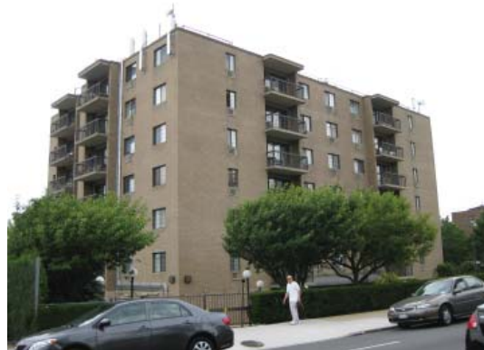
A six-story building on Metropolitan Avenue built between 1961 and 1997
