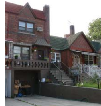
A two-story building on East 37th Street built before 1961
