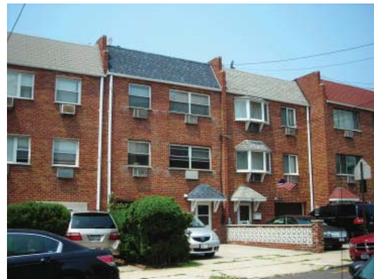
A three-story building on Monitor Street built between 1961 and 1997
