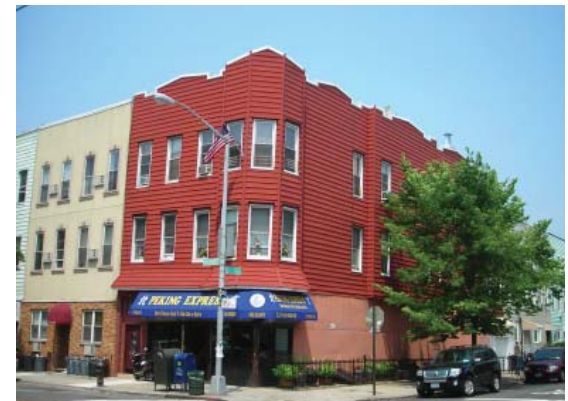
A three-story building on Nassau Avenue built before 1961
