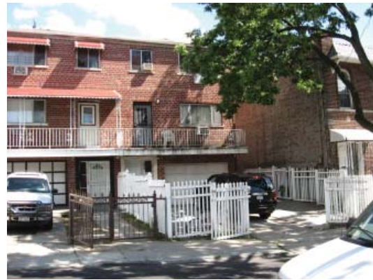
A three-story building on Baker Avenue, built between 1961 and 1997
