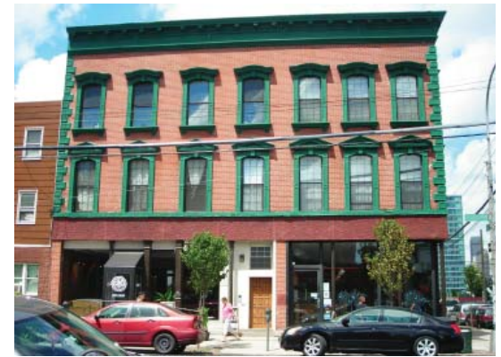
A three-story building on Vernon Boulevard built before 1961
