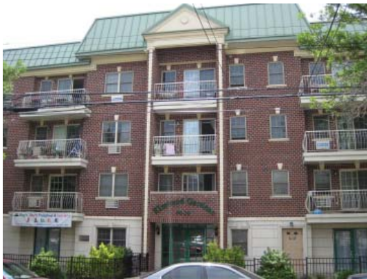
A four-story building on 55th Avenue built between 1998 and 2008
