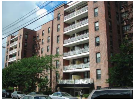
A six-story building on 37th Street built between 1961 and 1997
