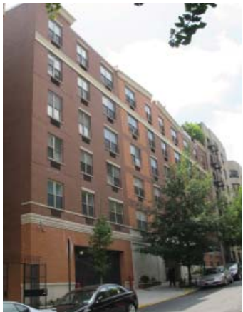
A seven-story building on West 187th Street built between 1998 and 2008
