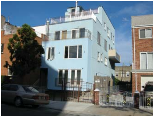
A four-story building of 37th Street built between 1998 and 2008
