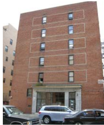
A six-story building on New York Avenue built between 1961 and 1997
