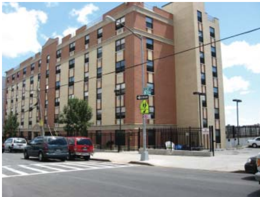
A six-story building on Jesup Avenue built between 1998 and 2008
