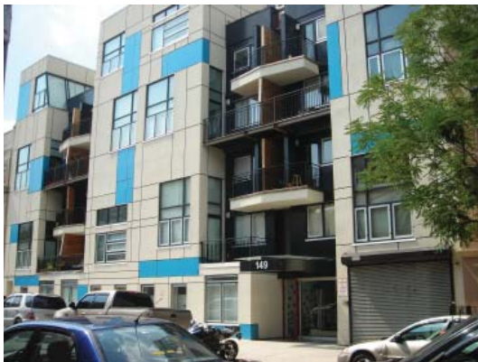
A six-story building on Huron Street built between 1998 and 2008
