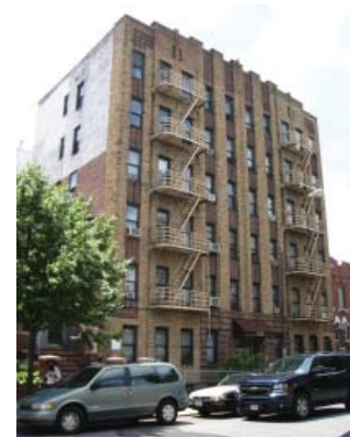
A six-story building on Carroll Street built before 1961
