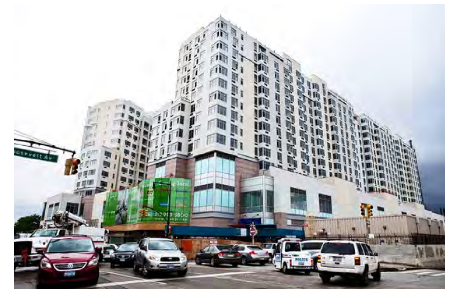
50+ Unit Building Complex on College Pt Blvd
