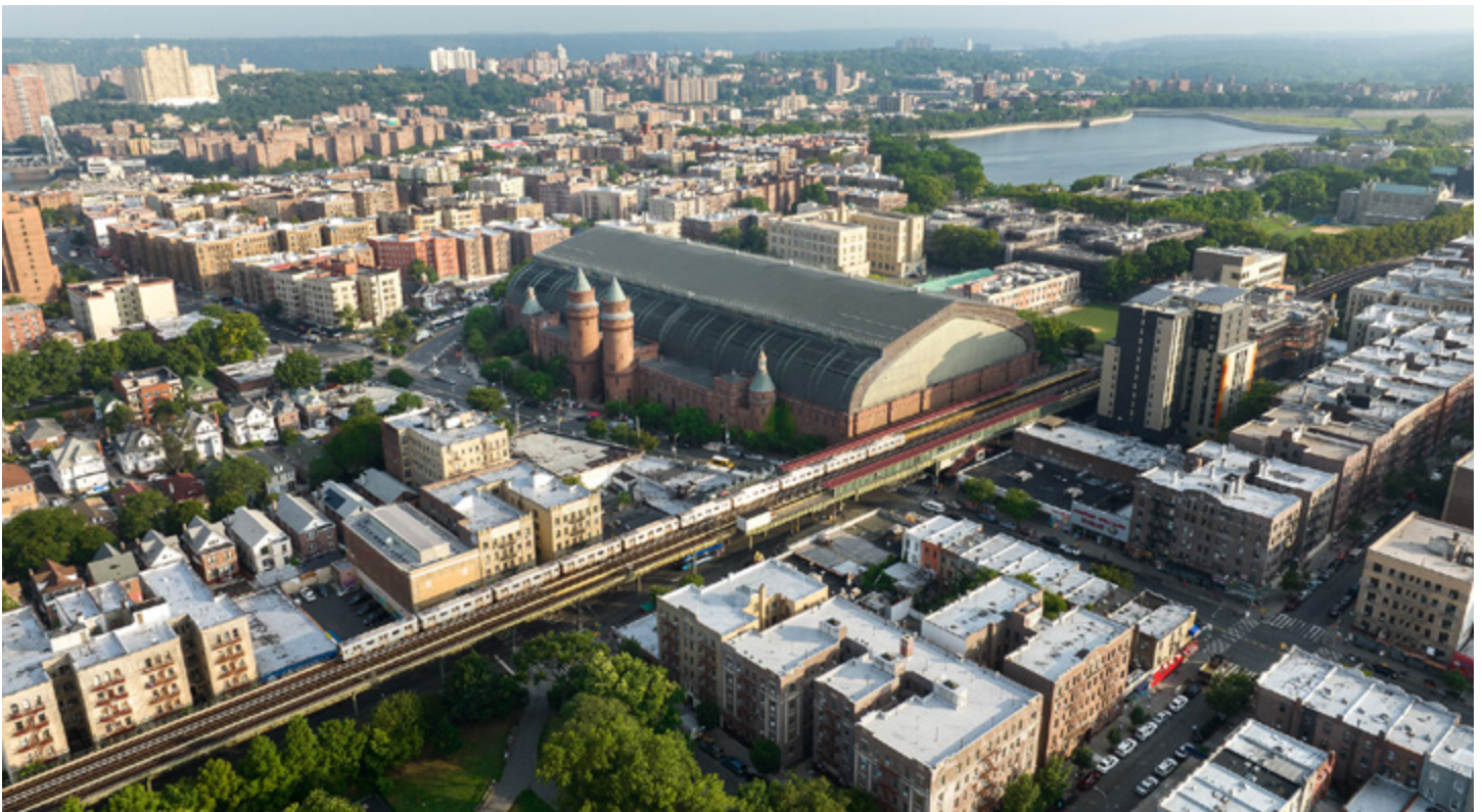
Kingsbridge Armory in The Bronx. Credit: NYCEDC
