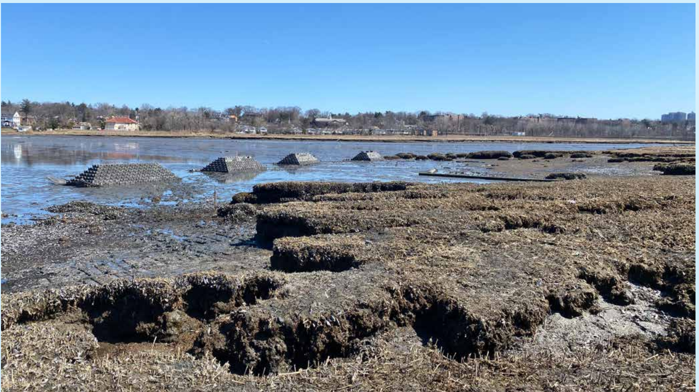
Above: Alley Creek living shoreline installation, Queens.
