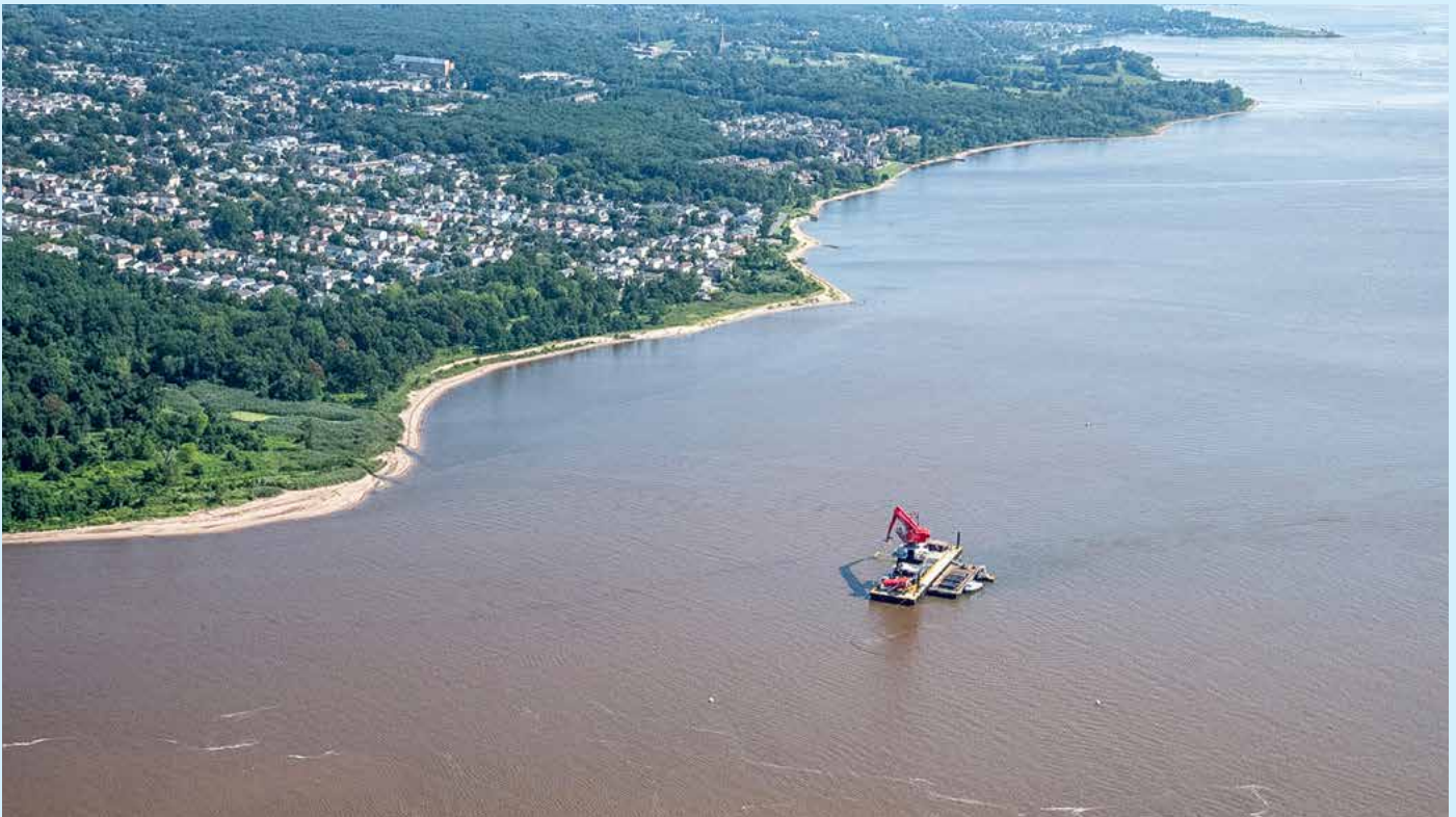
Above: Living breakwaters construction, Staten Island.
