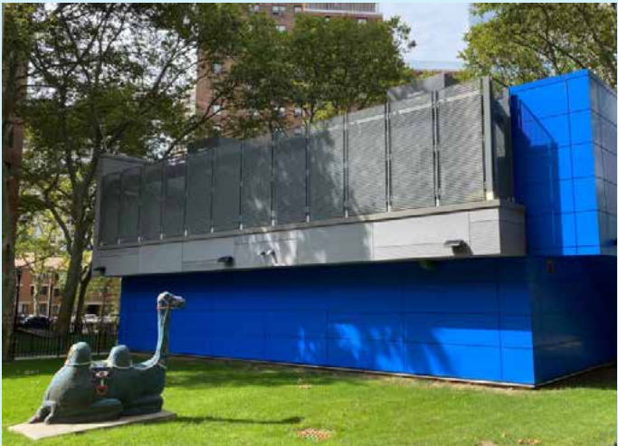
Elevated utility annexes serving NYCHA developments at LaGuardia Houses in Manhattan and Coney Island Houses in Brooklyn. Credit: NYCHA
