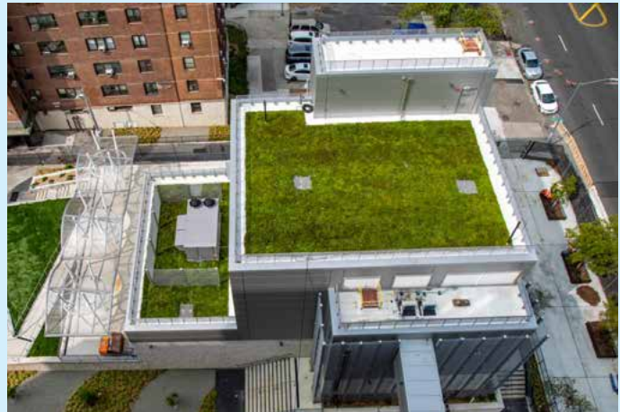
Elevated boiler building, with shade structures, community space, green roofs and site improvements serving multiple buildings at Coney Island Houses in Brooklyn Credit: NYCHA
