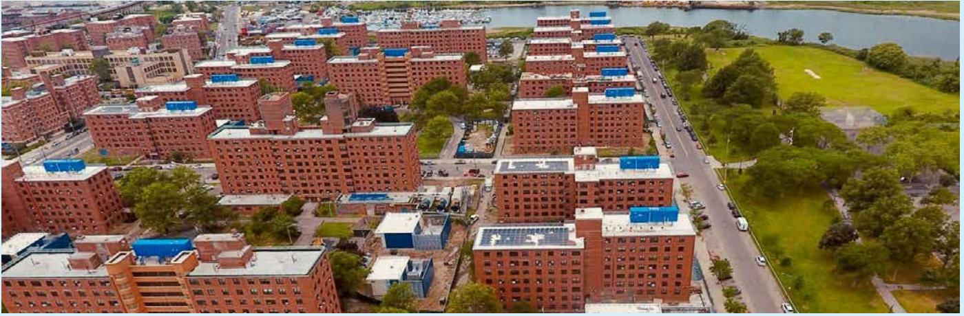
Generators and solar panels installed on the roof of each building of Ocean Bay Bayside Apartments in Arverne, Queens. Credit: NYCHA
