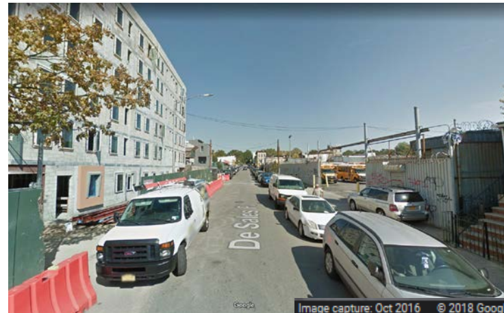
3. Bus parking and Riseboro affordable housing De Sales Place
