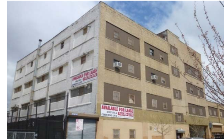
4. Multi-tenant manufacturing building 349 Suydam Street
