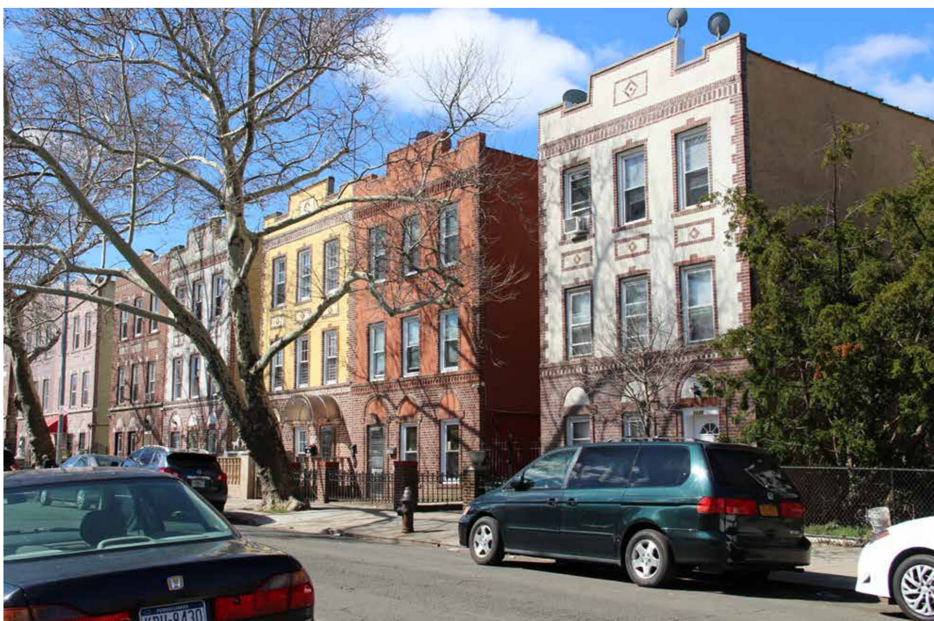
Photo: Street view showing low-rise residential developments
