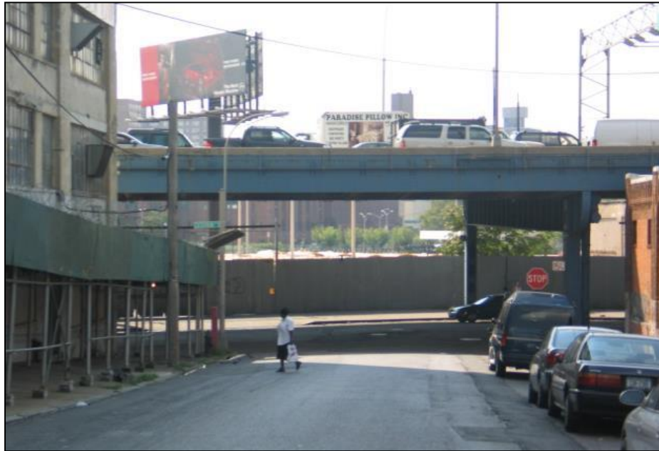
Elevated Major Deegan Expressway
