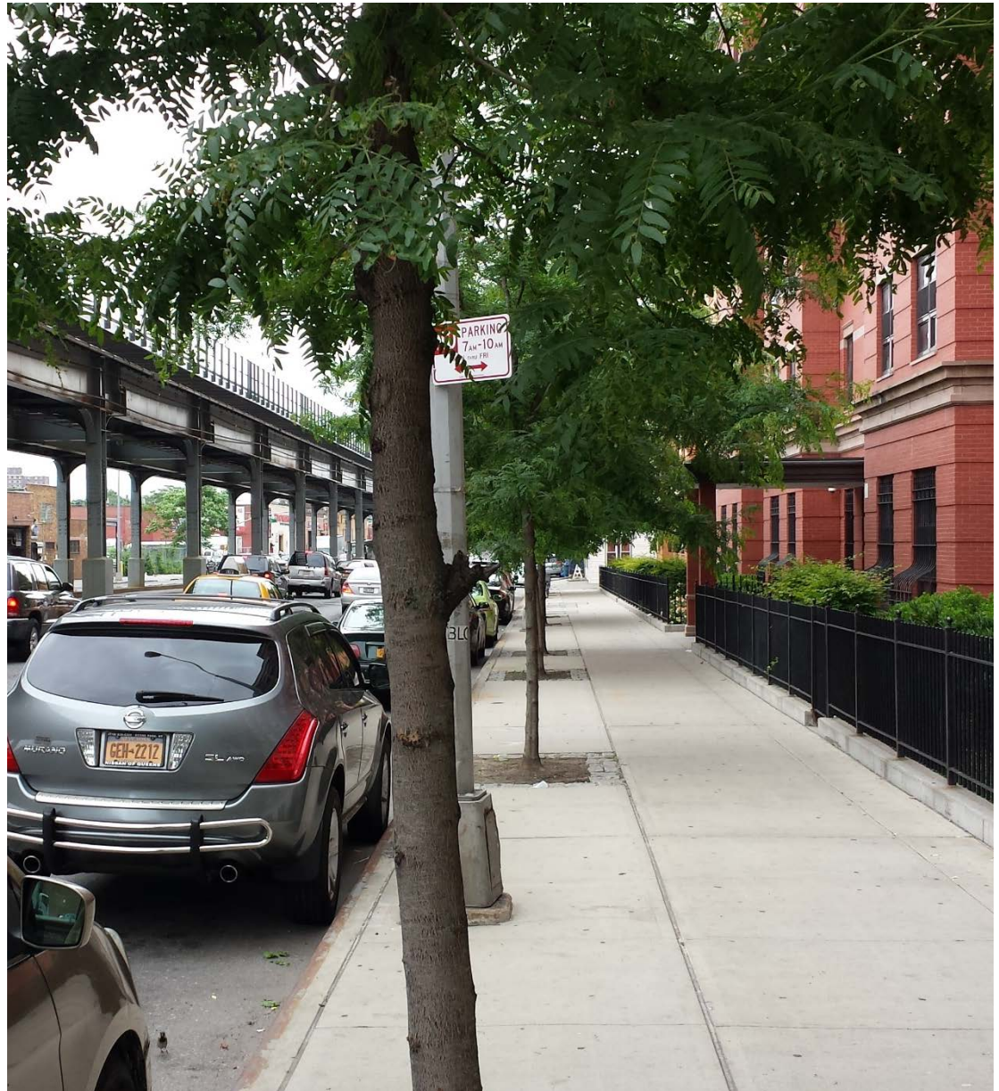
New construction on Atlantic Avenue near Buffalo Avenue
