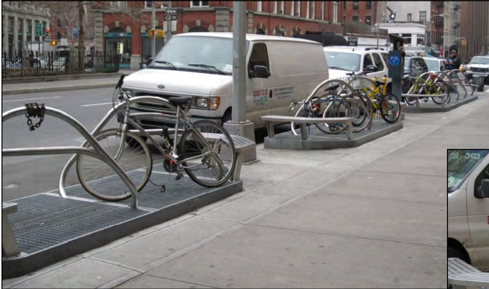
Elevated subway ventilation grates with built-in bicycle parking and sitting at West Broadway and Chambers Street
