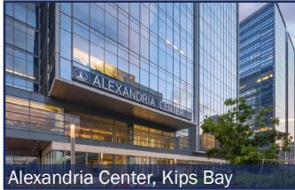
Alexandria Center, Kips Bay
