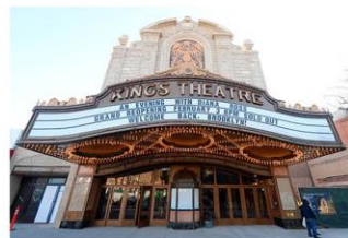
Kings Theatre 1027 Flatbush Ave, Brooklyn, NY 11226
