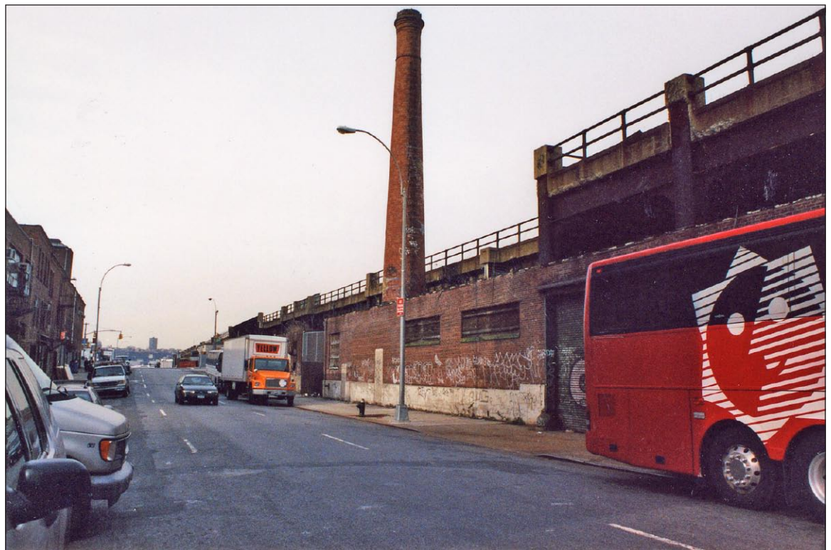
West 30th Street viaduct. View west toward Eleventh Avenue from West 30th Street trestle 2
