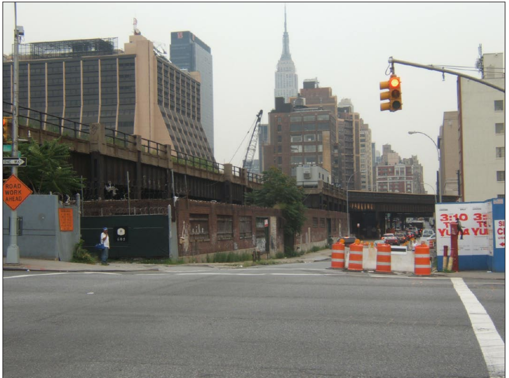
Rail spur along West 30th Street and trestle over West 30th. View east from Eleventh Avenue 1
