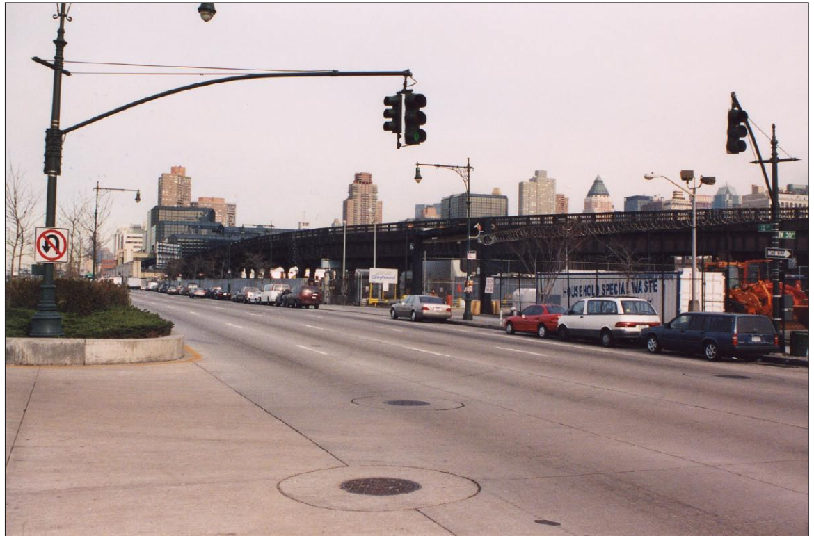
View of viaduct along Twelfth Avenue on Development Site. 5 View north on Twelfth Avenue from West 30th Street
