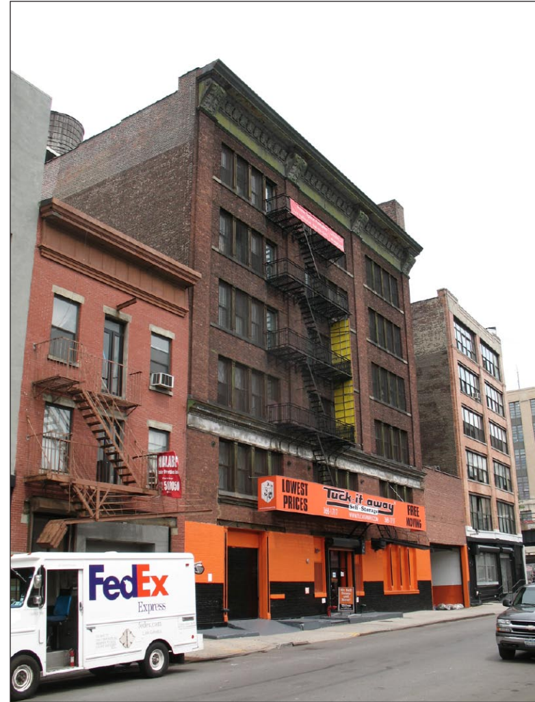
Charles P. Rodgers & Company Building, 517-523 West 29th Street 10
