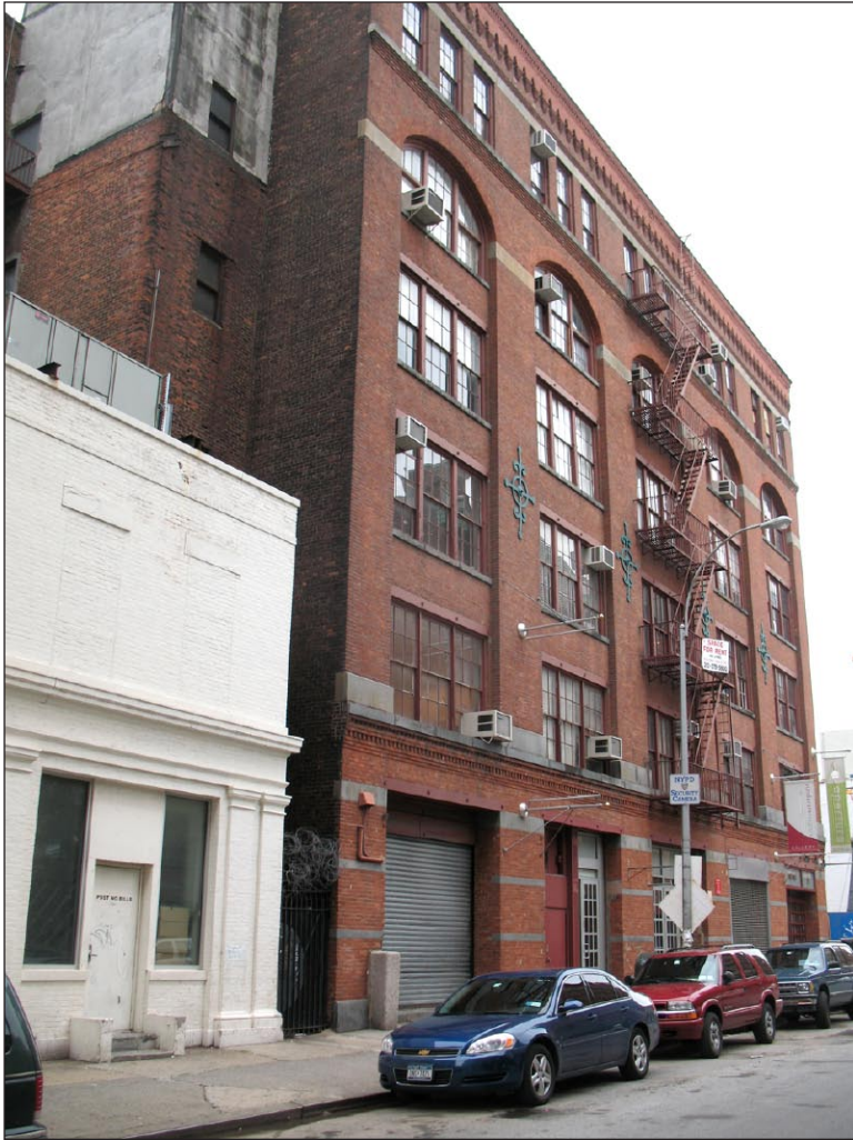
Former Berlin & Jones Envelope Company, 11 547-553 West 27th Street. View on West 27th Street
