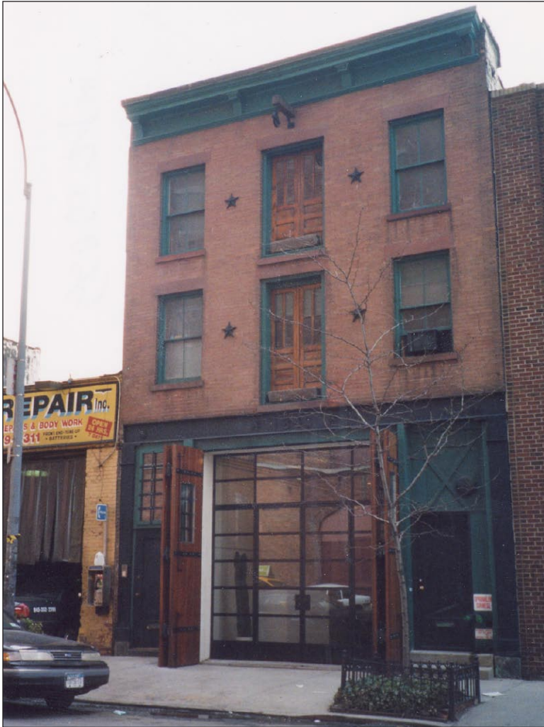
550 West 29th Street. View south 9
