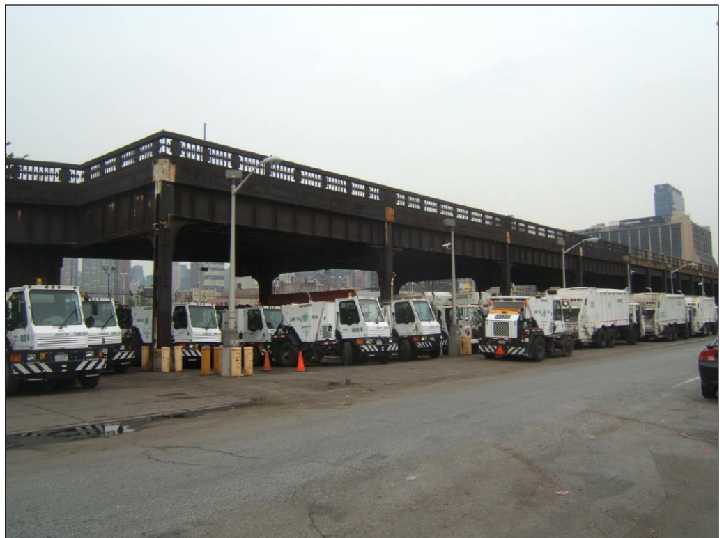
View of West 30th Street viaduct on Development Site. 4 View east towards Eleventh Avenue
