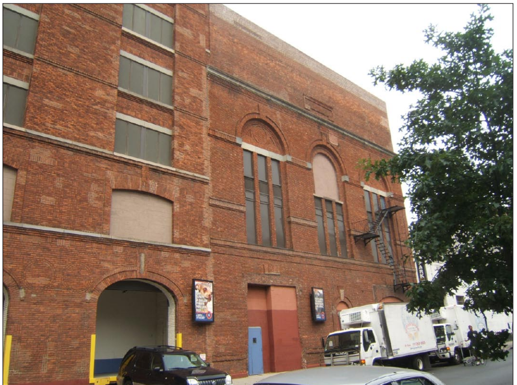
Garage of former W&J Sloane Warehouse, 541-547 West 29th Street. View north
