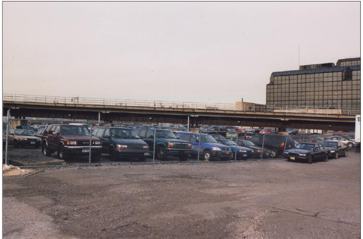
Curve in the viaduct as it moves from Twelfth Avenue to parallel West 34th Street. 6 View northwest from West 33rd Street
