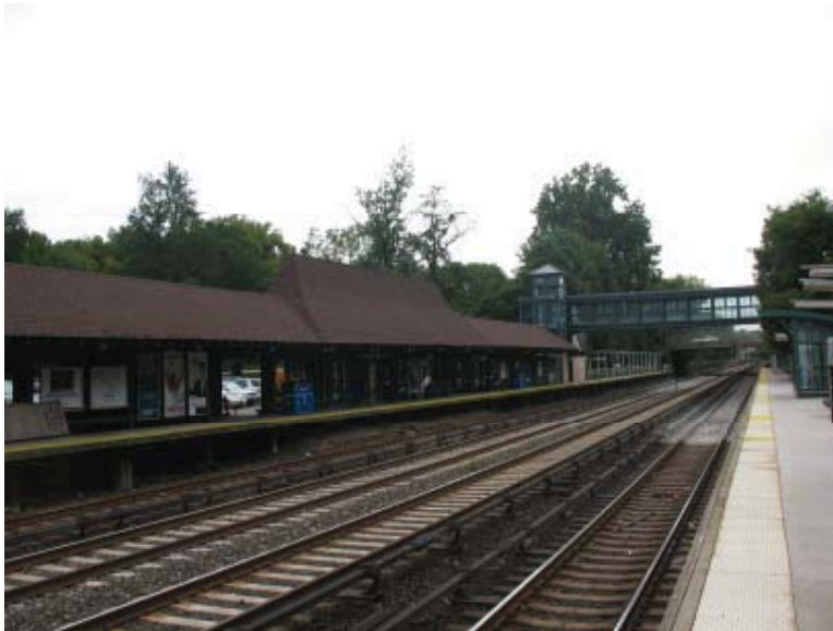
Resource #8: View looking southeast toward the station and platforms of the Metro North Railroad Botanical Garden Station, Botanical Square and Webster Avenue (November 2009).
