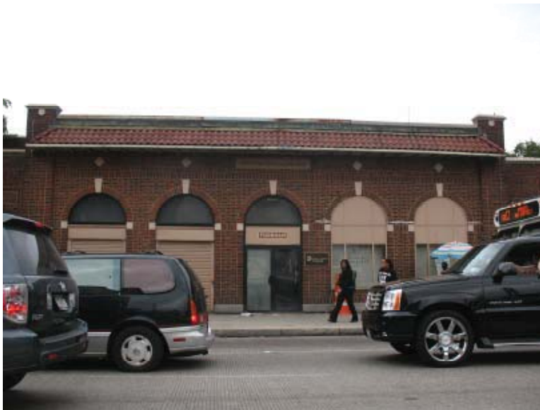
Resource #2: View looking north toward the Metro-North Railroad Fordham Road Station, East Fordham Road and Webster Avenue.
