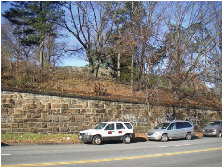
(11) Southeastern extent of Woodlawn Cemetery (series of retaining walls and perimeter trees), as viewed from Webster Avenue, looking northwest.
