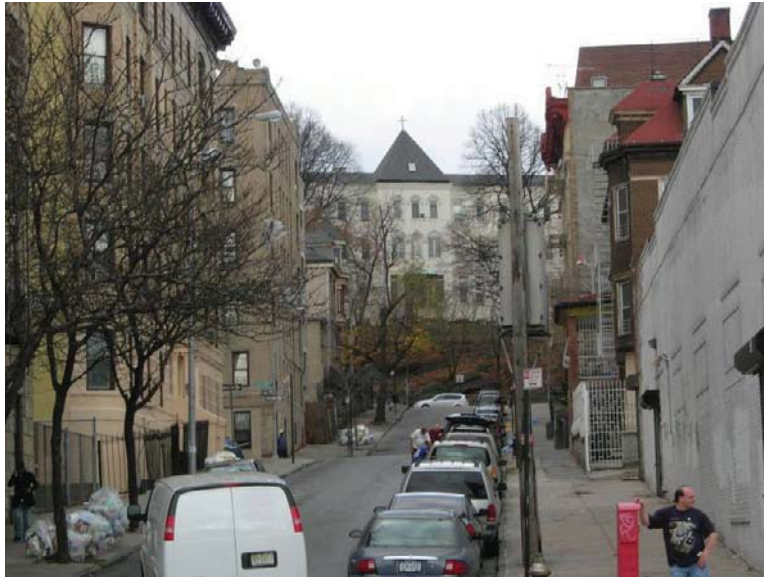
(7) Westerly view from Webster Avenue up East 199 th Street toward the Mount Saint Ursula Campus (main building visible in center of photo).
