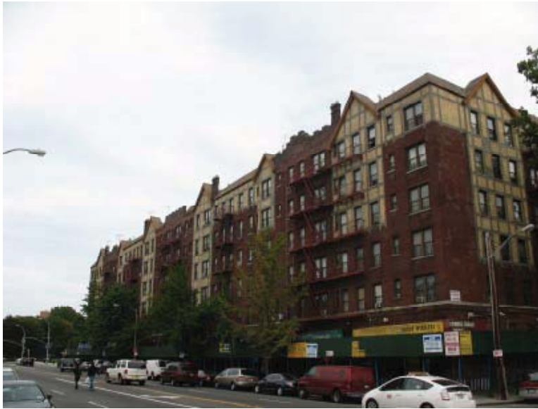
Resource #1: View looking northeast toward the Botanical Garden Arms, 2988-2990 Webster Avenue.
