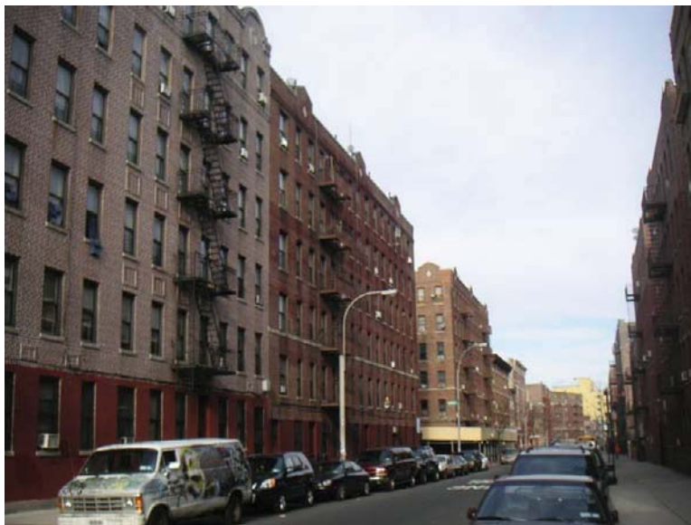
(2) Six-story apartment buildings in Norwood neighborhood.
