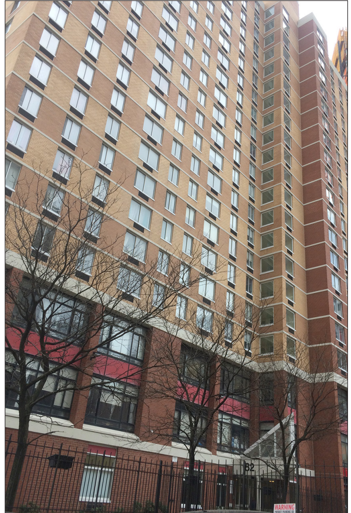
Looking west from Rutgers Slip Open Space to urban structure exterior ecological community adjacent to 82 Rutgers Slip 2
