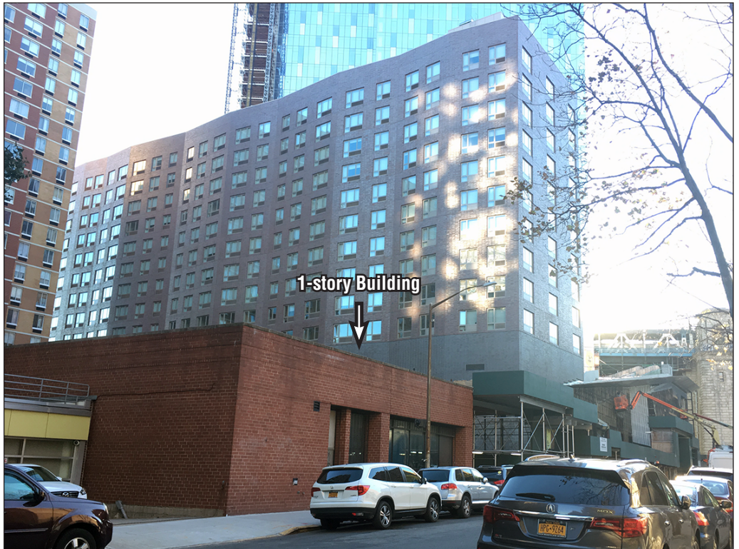
View southwest from Cherry Street to one-story building on Site 4 (4A/4B) 1
