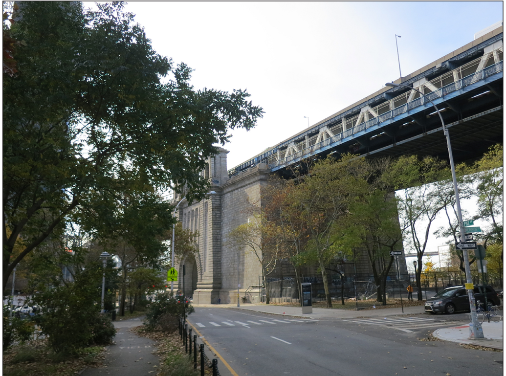
View of the Manhattan Bridge from Pike Slip 8
