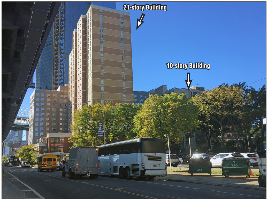
View northwest to Site 4 (4A/4B) from South Street 3
