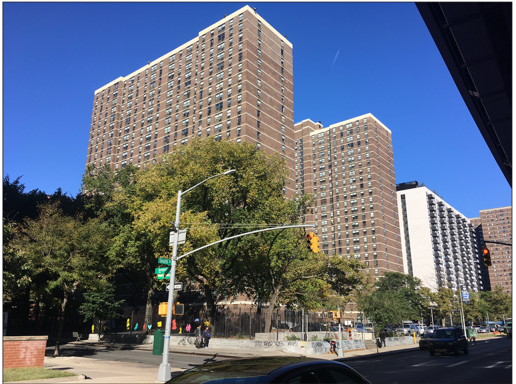
View northeast to Site 5 from Rutgers Slip and South Street 5
