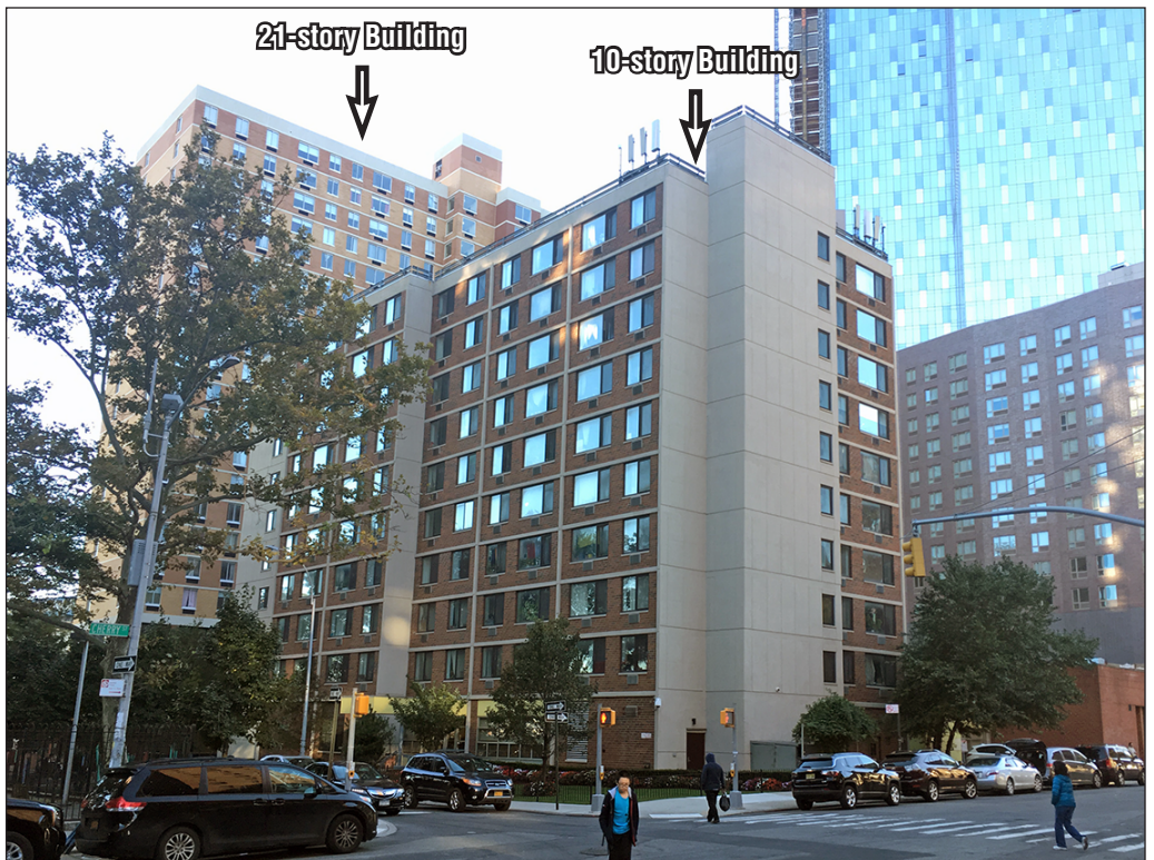
View southwest to Site 4 (4A/4B) from Cherry Street and Rutgers Slip 2
