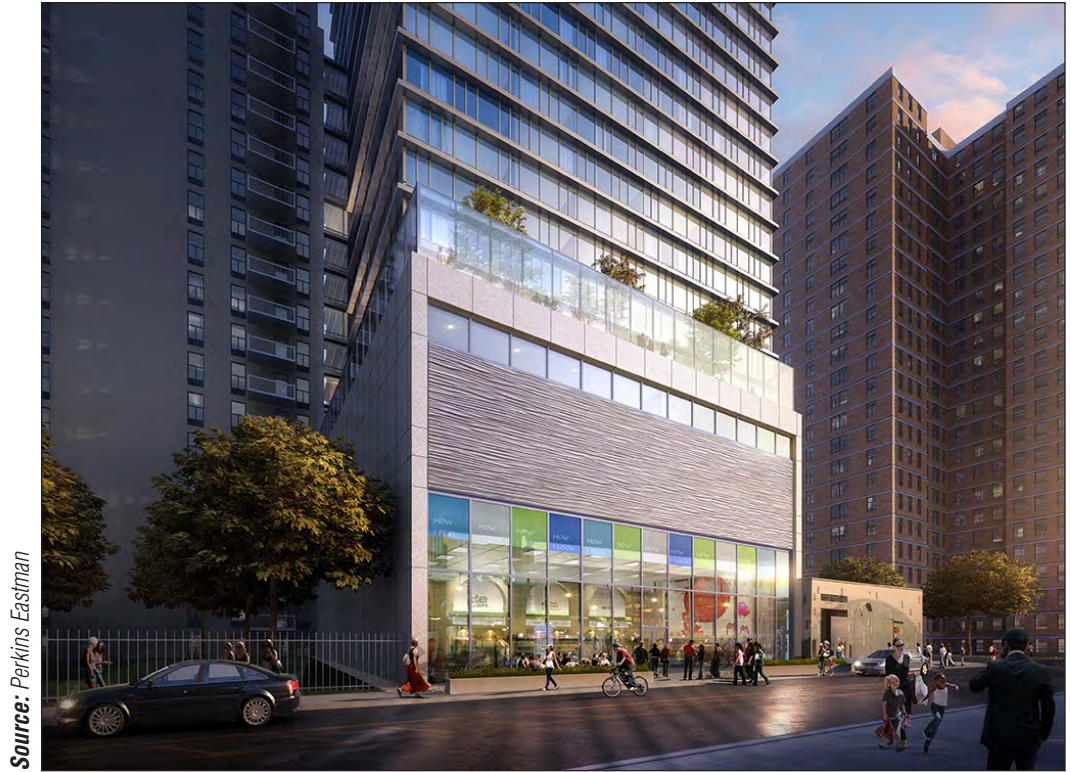
View northeast on South Street
