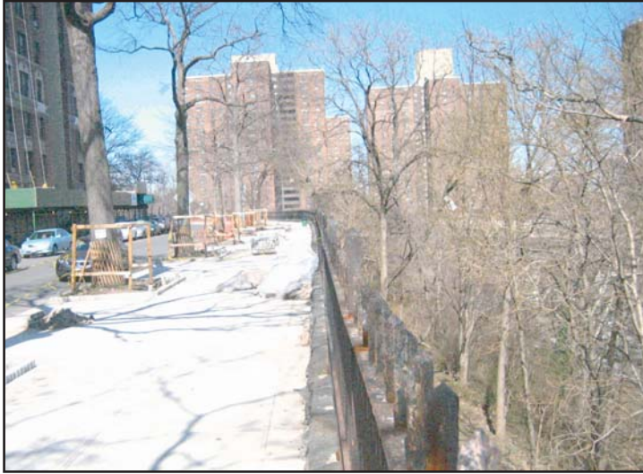
Topography - View from Edgecombe Avenue looking northeast, illustrating steep change in grade between Edgecombe Avenue and Jackie Robinson Park below (to the right). Polo Grounds Houses visible in background.
