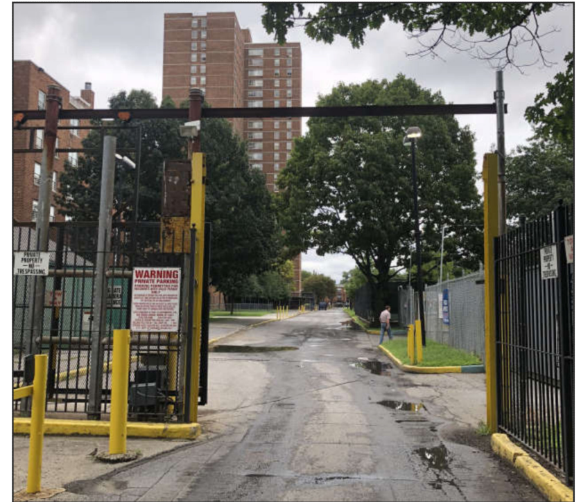
View from Lafayette Avenue between Leland and Underhill Avenues, looking south towards gated vehicle entry to Stevenson Commons.
