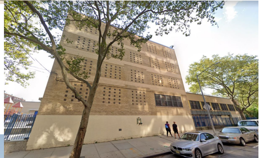
2. Eastern facade of the S/NR-eligible P.S. 100 along Thieriot Avenue.
