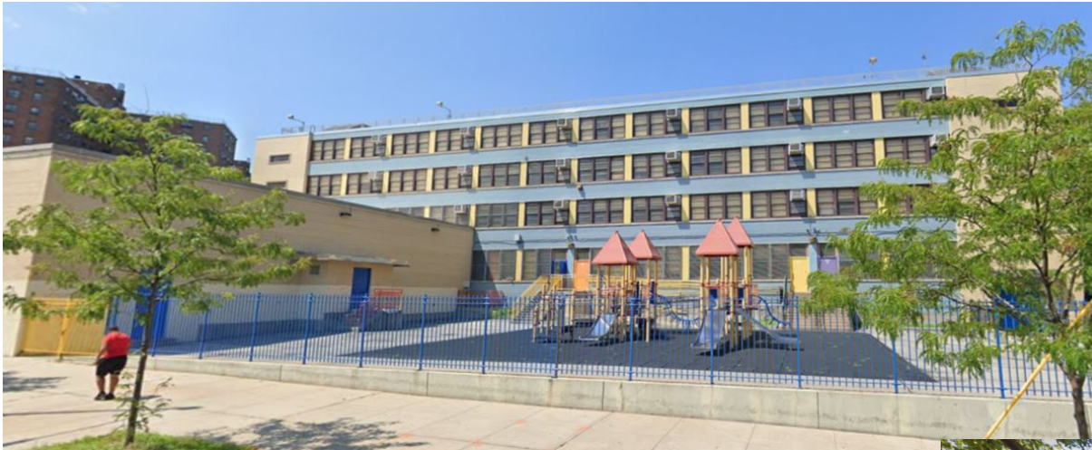
1. Southern facade of the S/NR-eligible P.S. 100 from Lafayette Avenue, with the Monroe Houses in the background.
