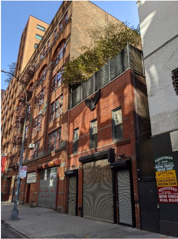
Photo captured by VHB October 6, 2020
