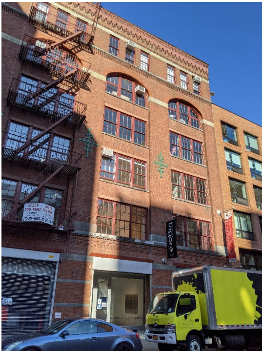
Photo captured by VHB October 6, 2020
