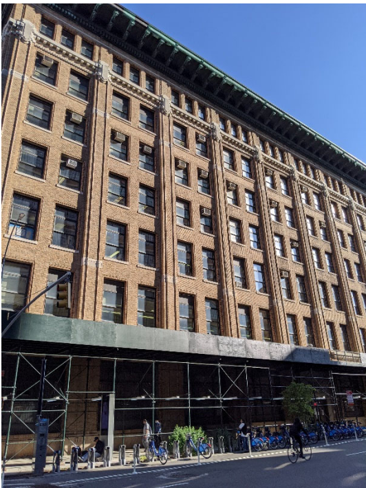
Photo captured by VHB October 6, 2020
