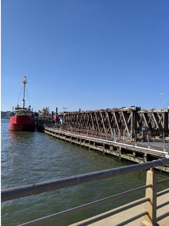
Photo captured by VHB October 6, 2020
