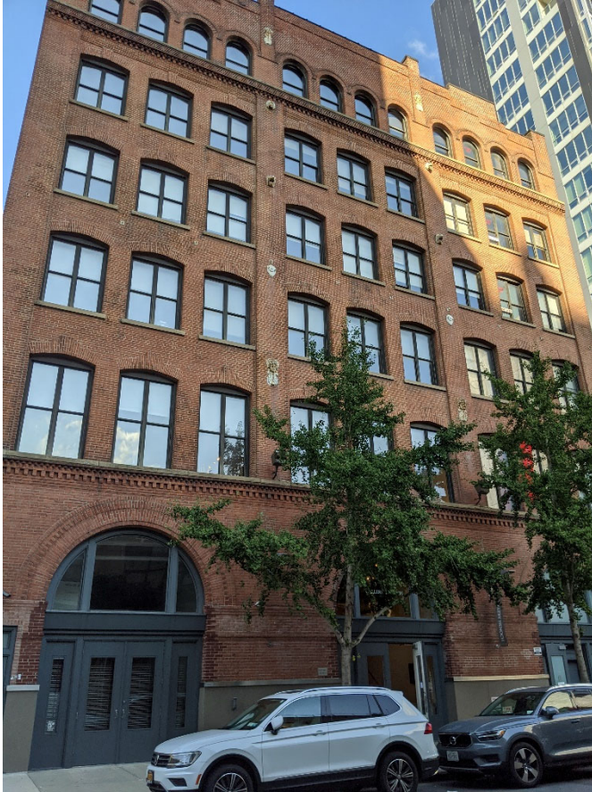
Photo captured by VHB October 6, 2020
