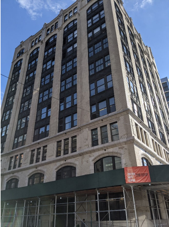
Photo captured by VHB October 6, 2020
