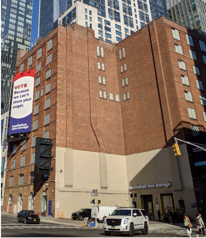
Photo captured by VHB October 6, 2020
