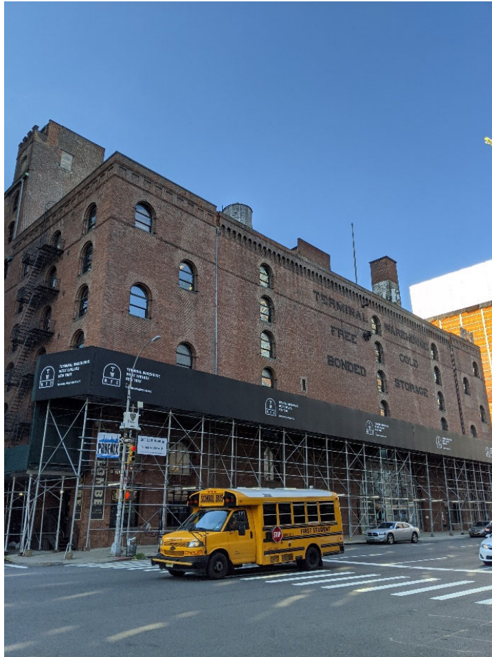
Photo 3 Terminal Warehouse Building
