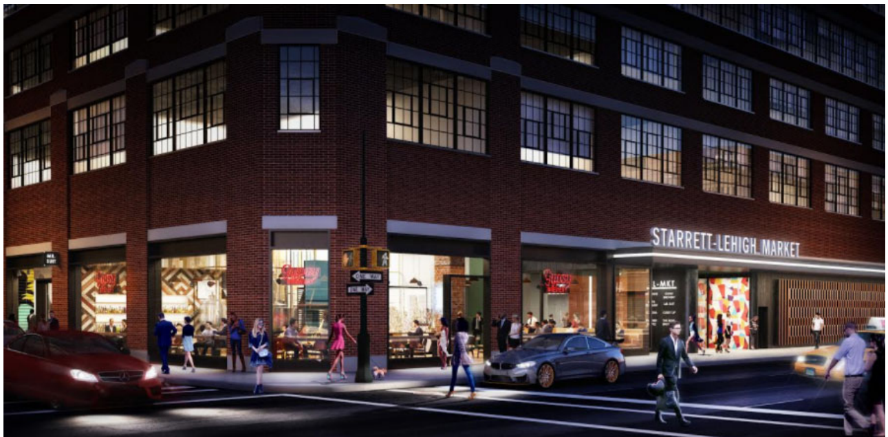
Photo 2 No-Action Condition: Starrett-Lehigh Building
