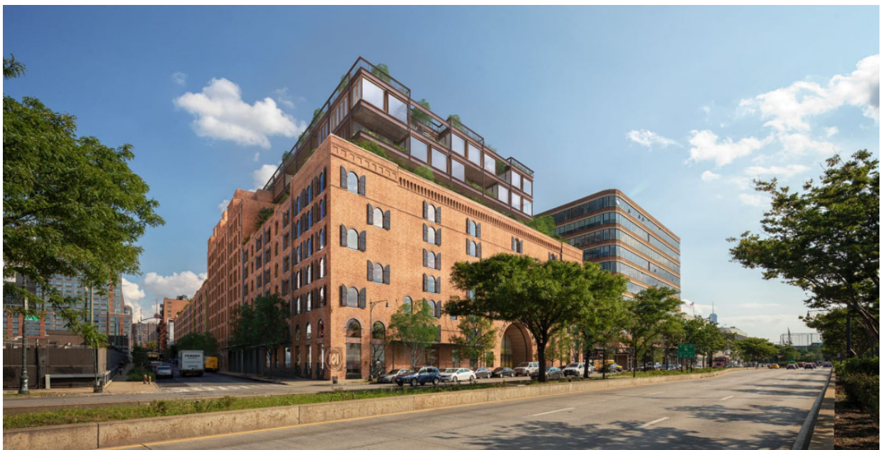
Photo 4 No-Action Condition: Terminal Warehouse
