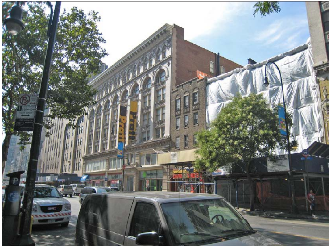
View southeast to south side of West 14th Street near Seventh Avenue 27
