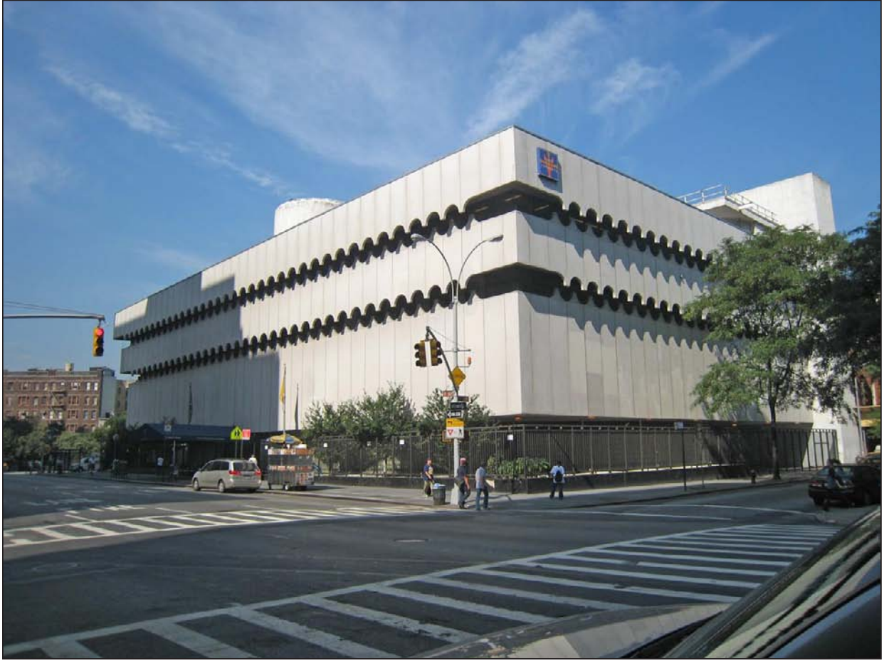
O'Toole Building — 20-40 Seventh Avenue (North and East Facades) 13
