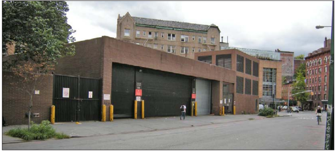
Materials Handling Facility (West 12th Street Facade) 10
