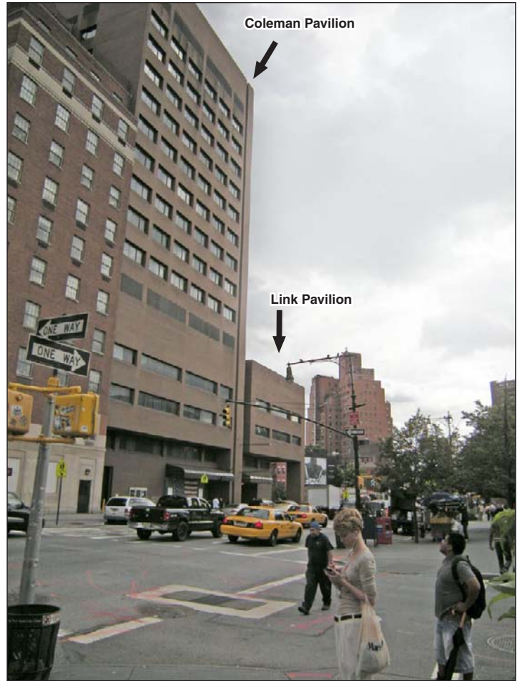
View south on Seventh Avenue from West 12th Street 14
