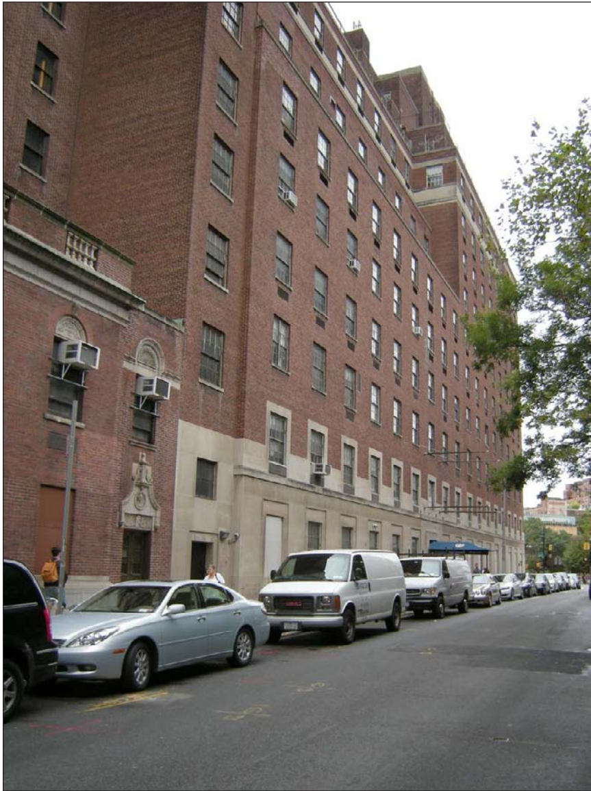
Smith/Raskob Buildings - West 12th Street Facade 3
