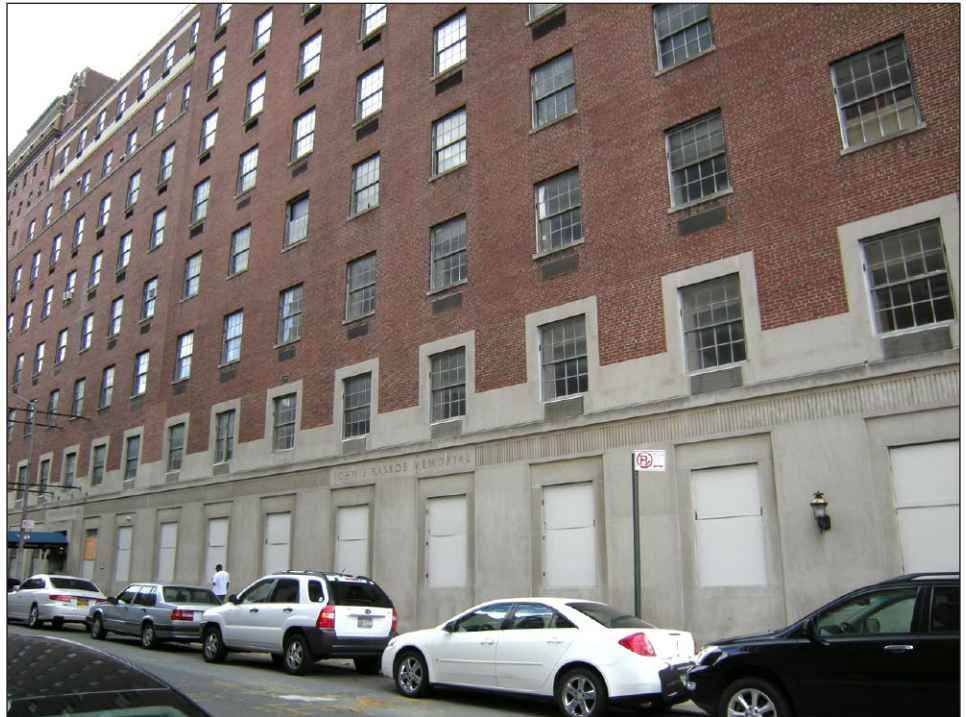
Smith and Raskob Building, view southeast on West 12th Street
