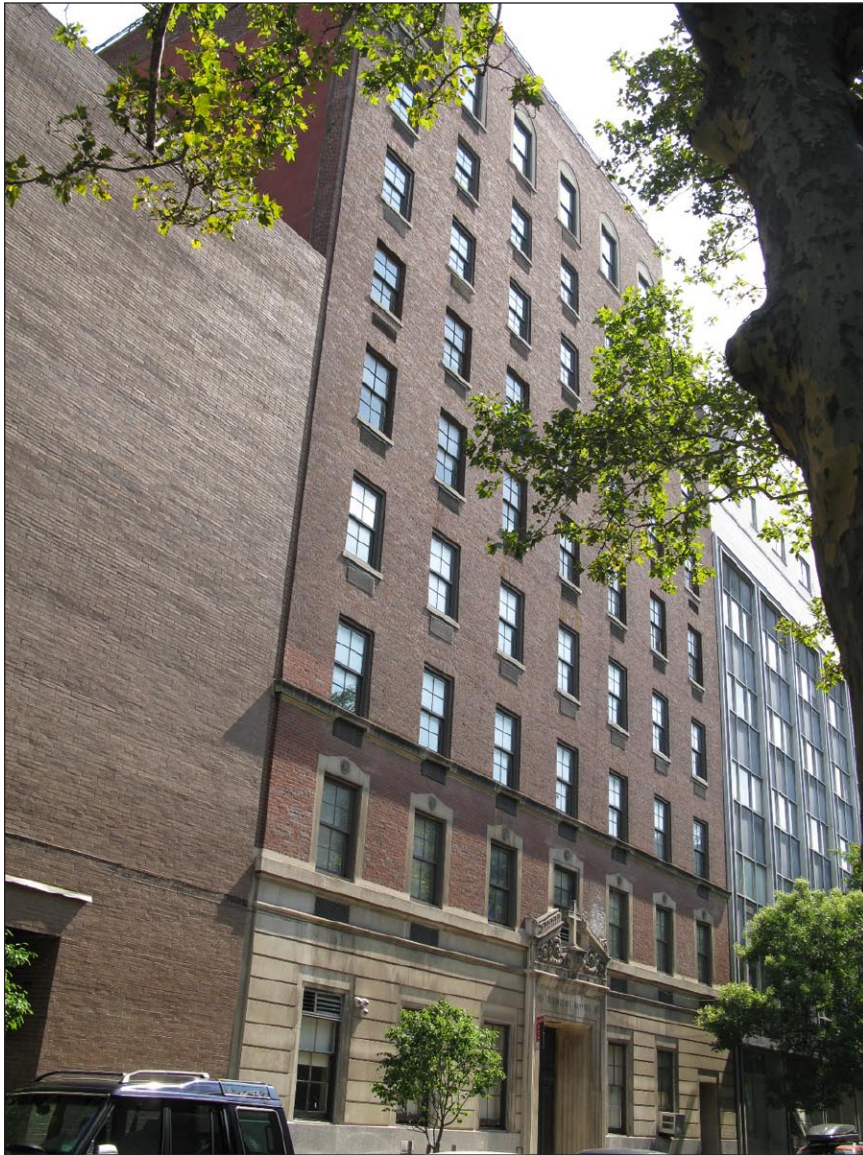
Spellman Pavilion, view northeast on West 11th Street 8
