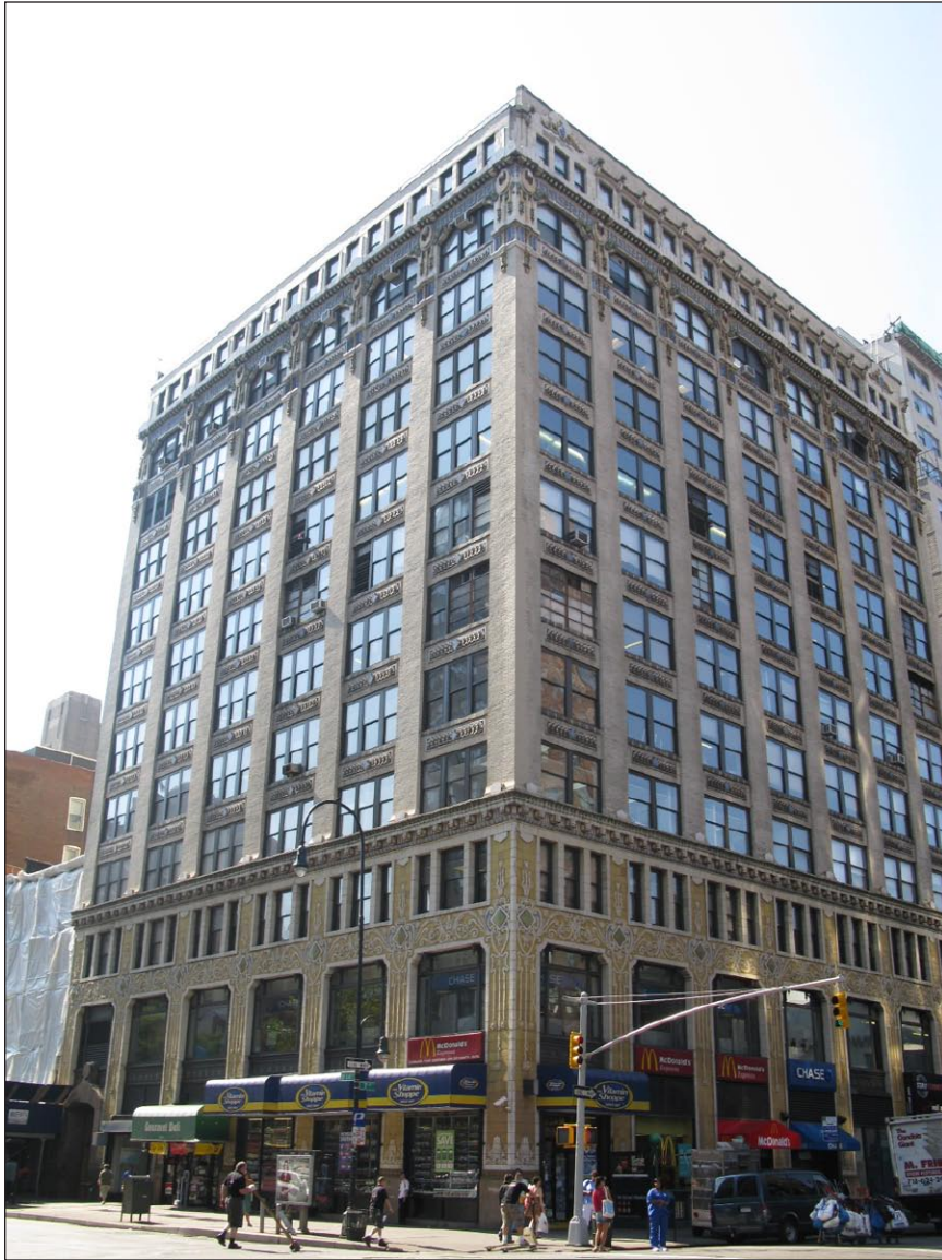
12-story Loft Building, 154 West 14th Street 20
