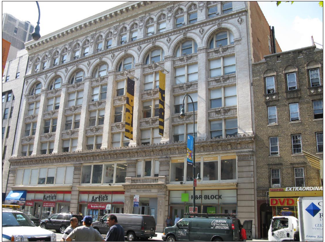
Pratt Institute Building, 138-146 West 14th Street 19
