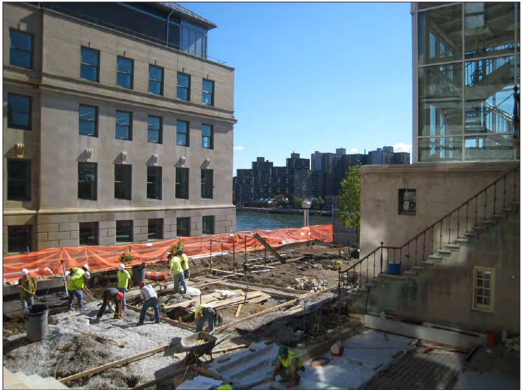
Looking northeast at a portion of the laboratory building site west of the FDR Drive
