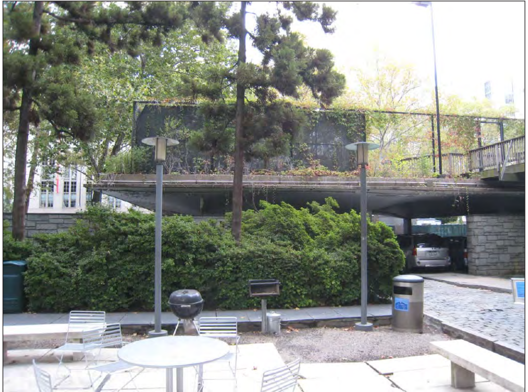
Looking north at the existing parking structure on the proposed recreation building site 3
