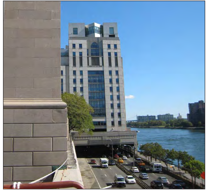
View north over the FDR Drive from near the Flexner Hall Extension 3
